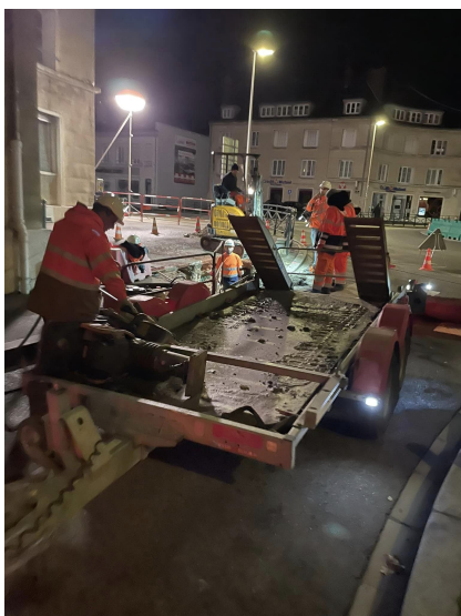
INTERVENTION NOCTURNE CANALISATION
